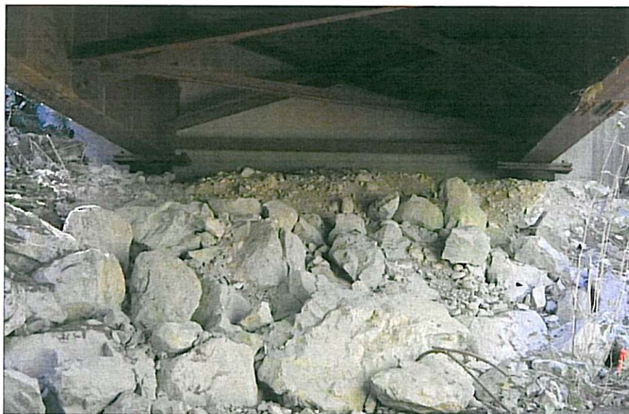
CK-2218 left abutment
