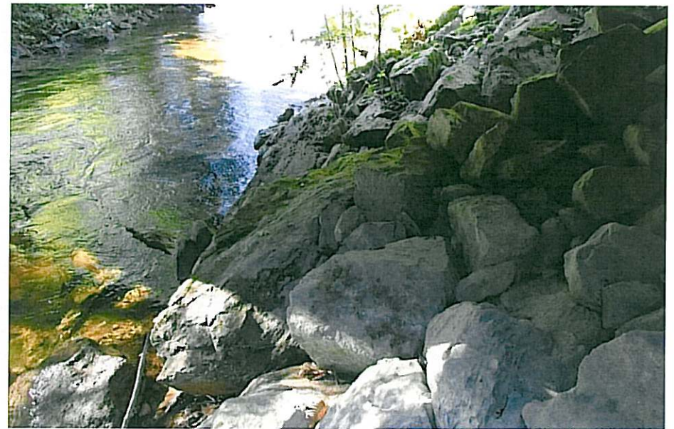
CK-2218 right abutment
